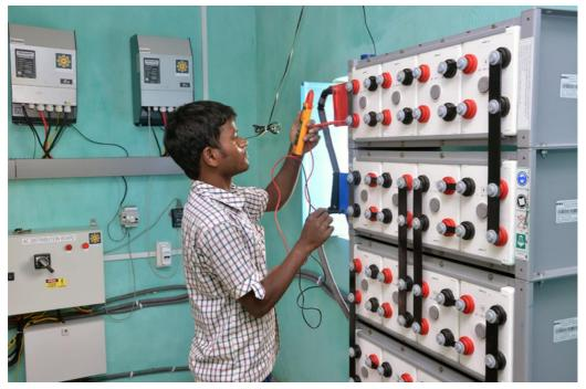
Mini-grid plant operator checks battery charge in mini-grid power house Source: Mlinda, 2019
