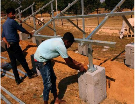
Local workers installing the framing for photovoltaic (PV) solar panels Source: Mlinda, 2019
