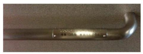
Figure 5-25: Handrail with Braille Information Panel
